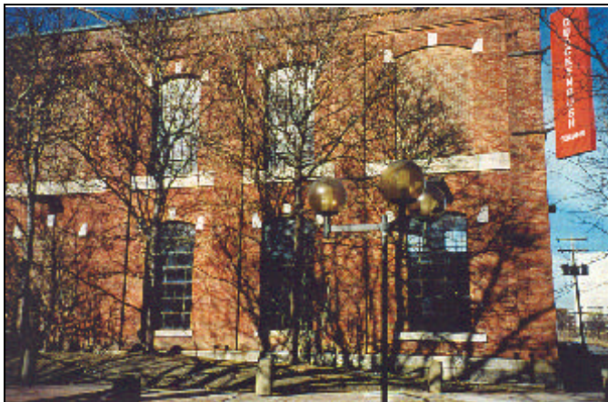
The historic Quackenbush Pump House is now home to the C.H. Evans Brewing Company Restaurant, "Albany Pump House".
